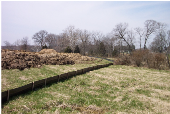
Example – Silt Fencing
